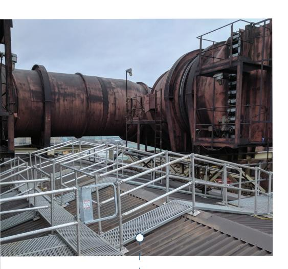
The RoofWalk system is designed to create a sure-footed walkway on your rooftop. This fully customizable platform made from non-slip materials and is installed above the roof membrane ensuring no damage is being done while it in use. Utilizing our counterweighted baseplates and RoofGuard rails, this system can be tailored to any flat roof application, providing safer access to any workspace by eliminating slipping and fall hazards.
