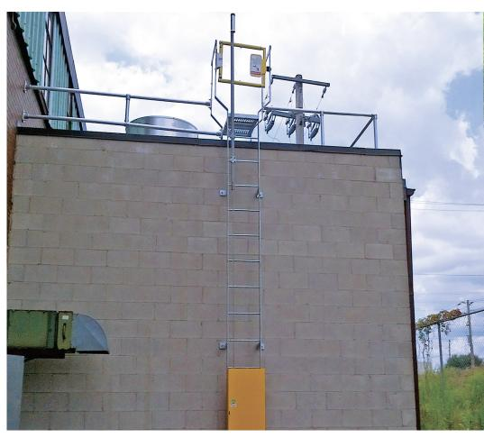
When you have created a regular access point to your roof or an elevated platform, you have created an unprotected leading edge. LadderGuard solves this potential problem with a system of guardrails designed to create an egress away from the leading edge of your rooftop.
