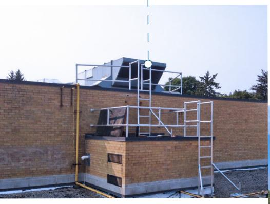
Ladder Series (LD) RoofStep systems help workers move from one level to another, and have guardrails on the upper side to help prevent a fall to the lower level.
