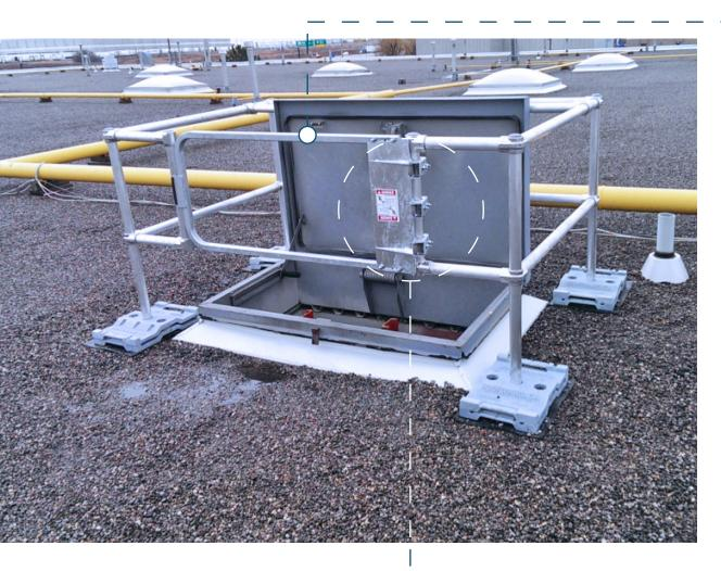
A standard spring-loaded gate ensures the gate always returns to the closed position, eliminating potential falls through the roof opening.
