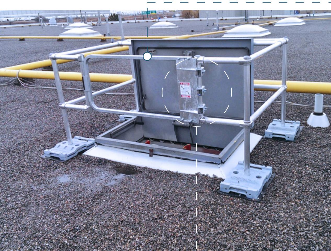
A standard spring-loaded gate ensures the gate always returns to the closed position, eliminating potential falls through the roof opening.
