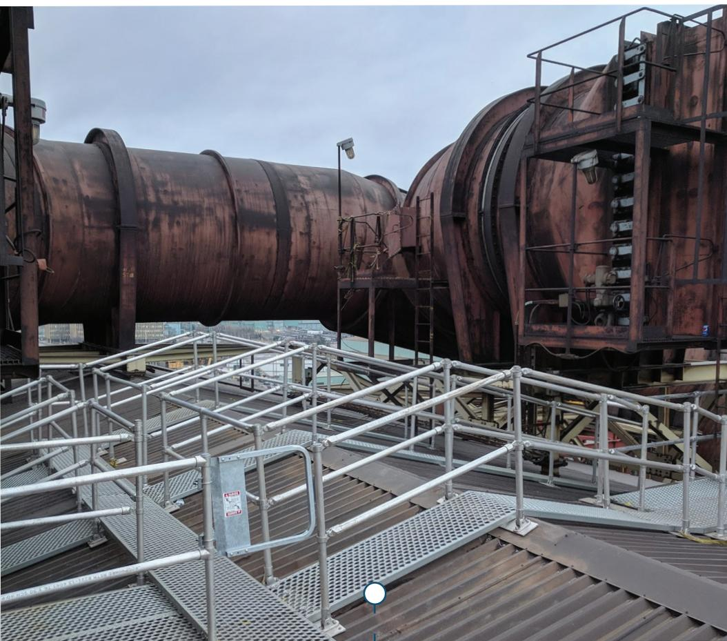
The RoofWalk system is designed to create a sure-footed walkway on your rooftop. This fully customizable platform made from non-slip materials and is installed above the roof membrane ensuring no damage is being done while it in use. Utilizing our counterweighted baseplates and RoofGuard rails, this system can be tailored to any flat roof application, providing safer access to any workspace by eliminating slipping and fall hazards.
