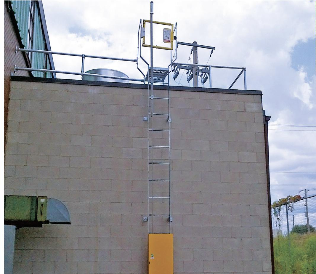
When you have created a regular access point to your roof or an elevated platform, you have created an unprotected leading edge. LadderGuard solves this potential problem with a system of guardrails designed to create an egress away from the leading edge of your rooftop.
